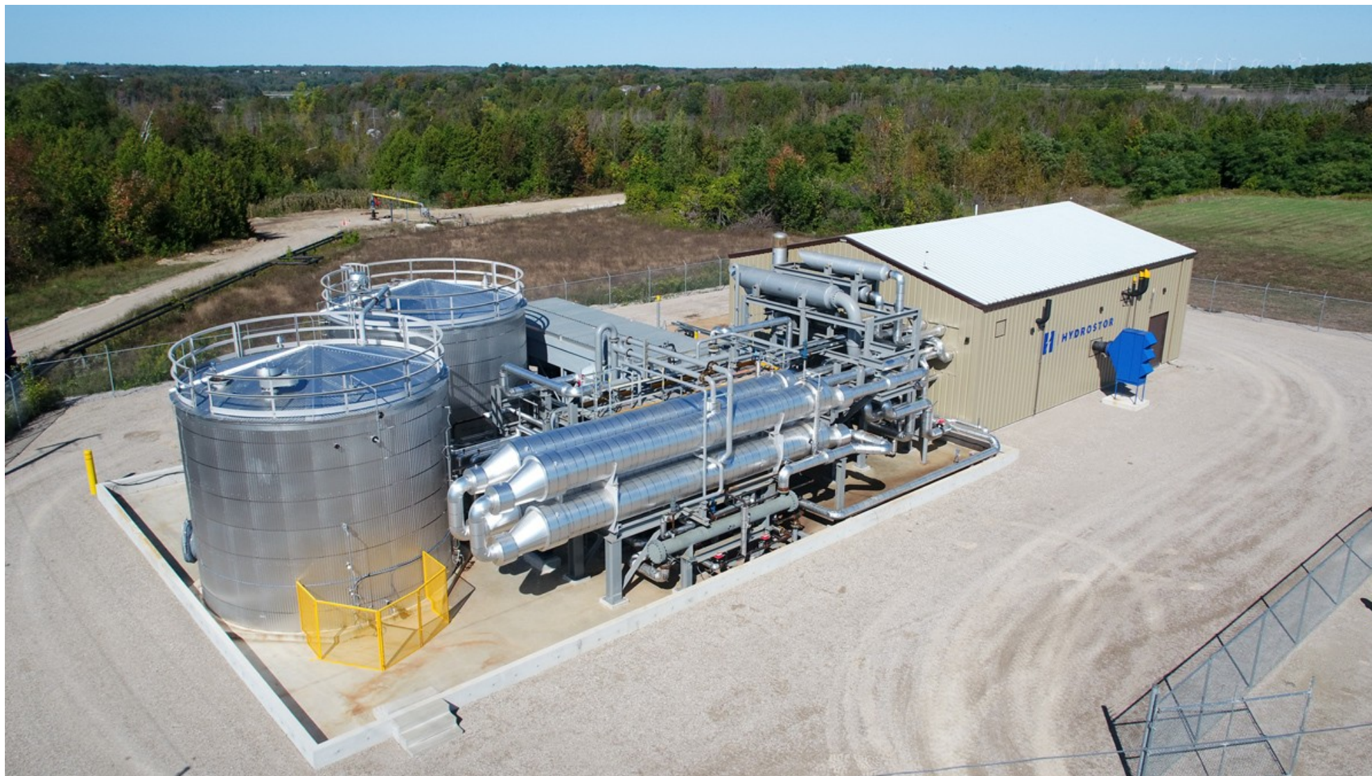
Compressed air energy storage (CAES) facilities, such as this Hydrostor facility, store energy generated by wind and solar power in the form of compressed air, sometimes storing it in underground caverns. Credit: Hydrostor
